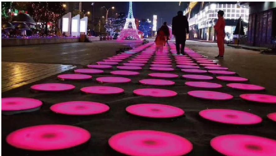
Round floor tile installation
